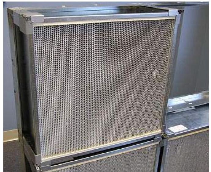
Figure 30: Properly Installed Filter Inside of the Frame
