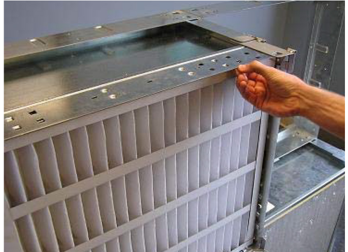
Figure 36: Installation of Prefilter into Frame
